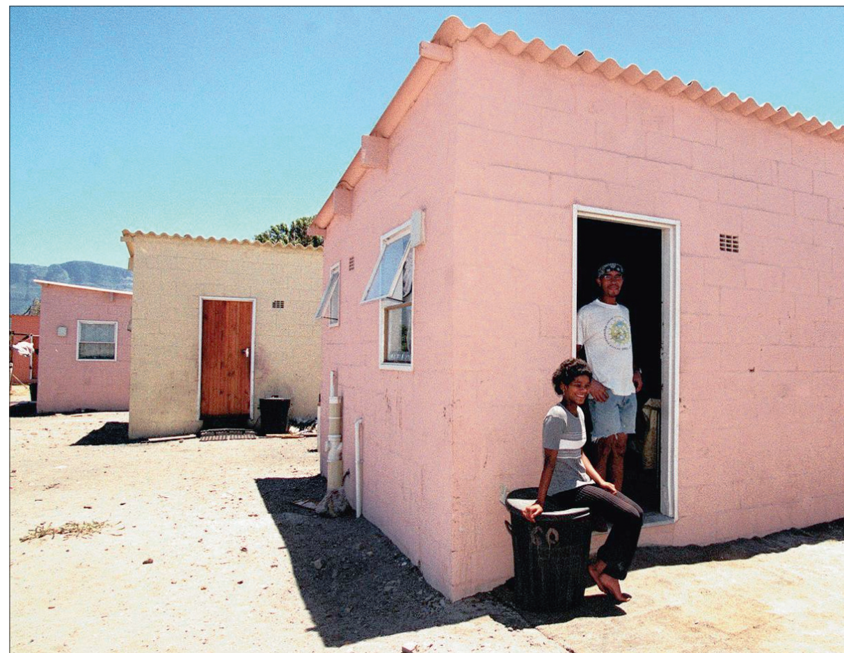
REPETITION: In the rush to build more and more small houses, it was forgotten that the programme was reinforcing the spatial logic of apartheid, says the writer.
